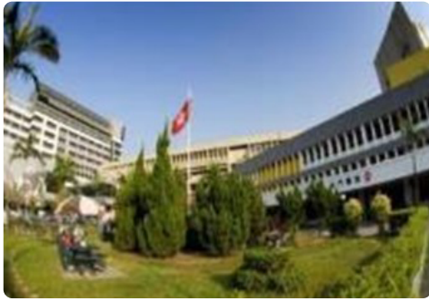
Tuen Mun Hospital (TMH)
